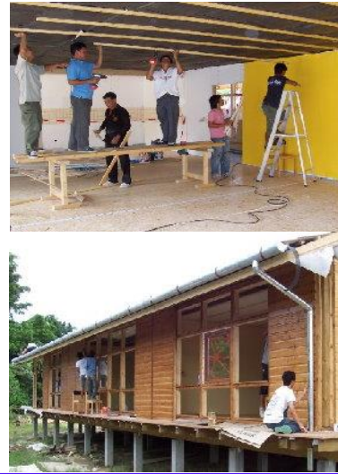
Kindergarten Rosenheim building site
